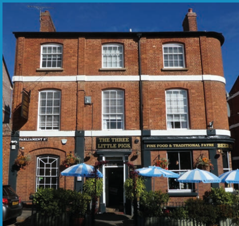
The pub is having a month-long renovation from early May.
