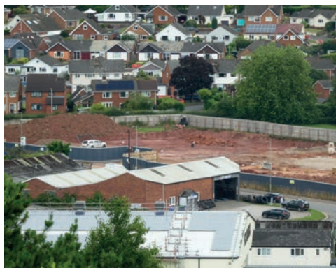
Groundworks for Lidl on former playing field
