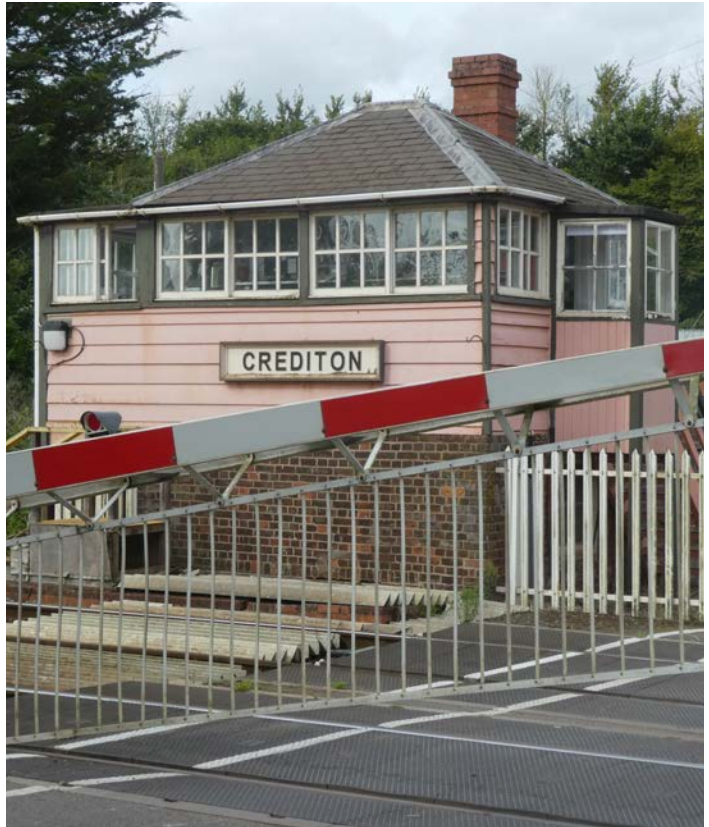
Level crossing gates rising in front of Crediton station's signal box
