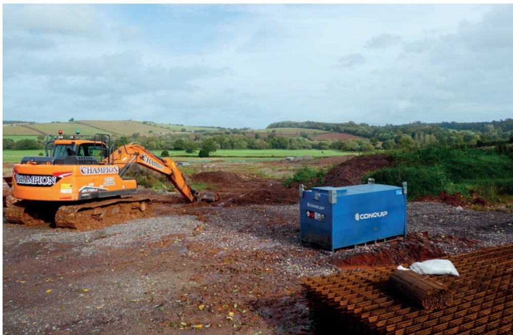
Digger, gravel, earth . . . work has started to build 257 homes at Pedlarspool
