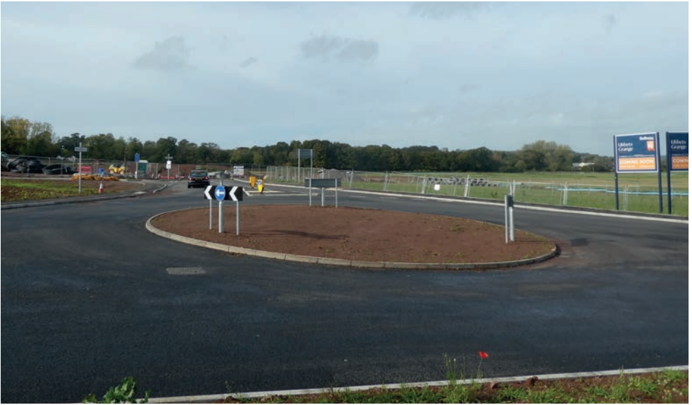
New roundabout providing access to new homes at Pedlarspool
