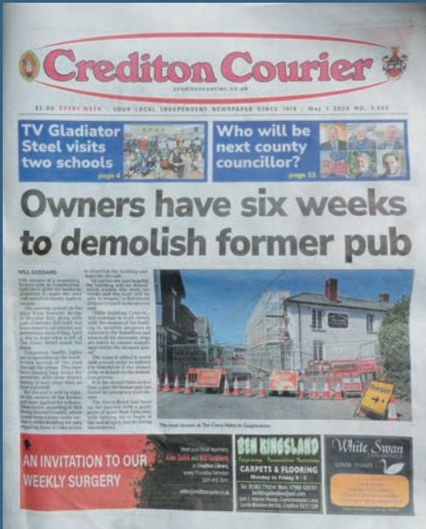
A recent Crediton Courier issue, reporting on major disruption in Copplestone caused by The Cross pub building on the verge of collapse. Villagers on foot and vehicles on the nearby A377 were severely affected
