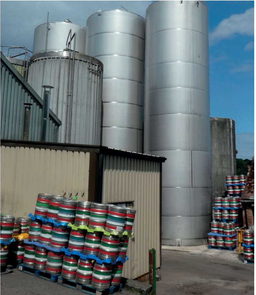
Bulk liquid storage (and casks) on Commonmarsh Lane
