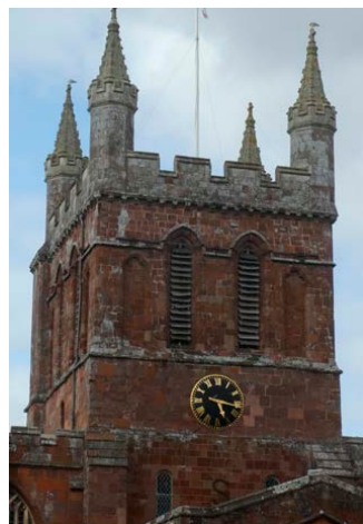
The bell chamber is in the uppermost part of the church tower, with louvred fenestration (wooden slats rather than glazed windows) on four sides to let the bells sound out in all directions
